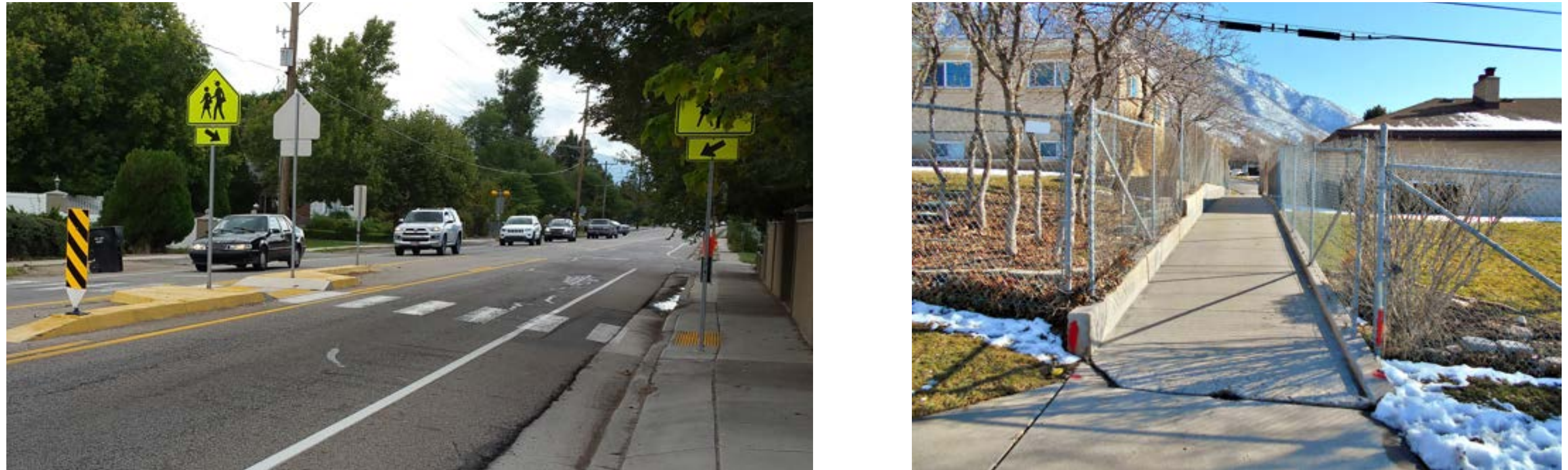
Examples of retrofit improvements that increase street connectivity in built-out areas include street crossing improvements (left) and a pedestrian pass-through (right)
