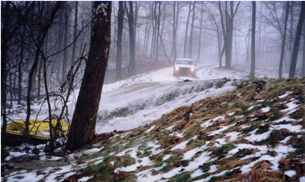
Figure 8. Overtopping Failure.
