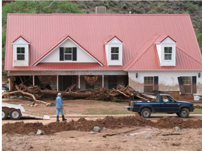
Figure 3. Flood Damage, Washington County, Utah .August 2007
