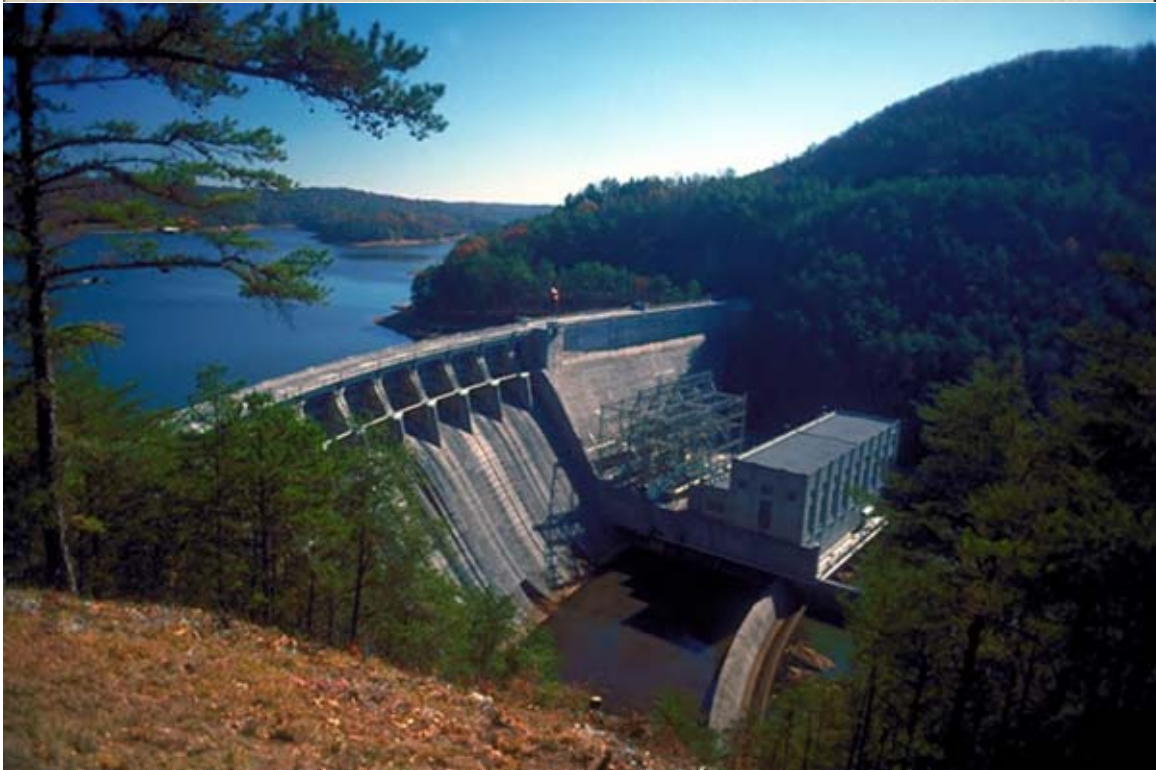
Figure 2. Concrete Arch Dam.
