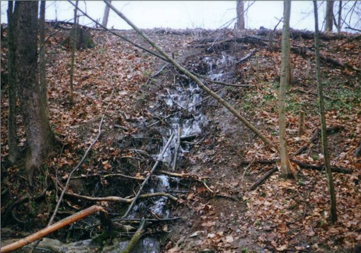
Figure 7. Piping Failure
