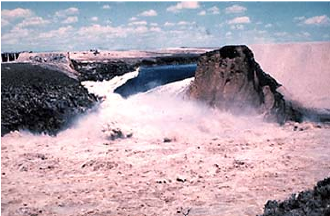
Figure 14. Teton Dam Failure.
