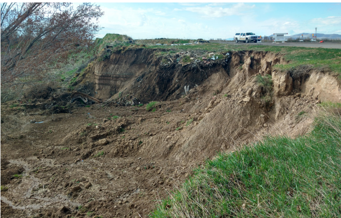
Image: Box Elder County landslide above development 2017. BEC Emergency Management
