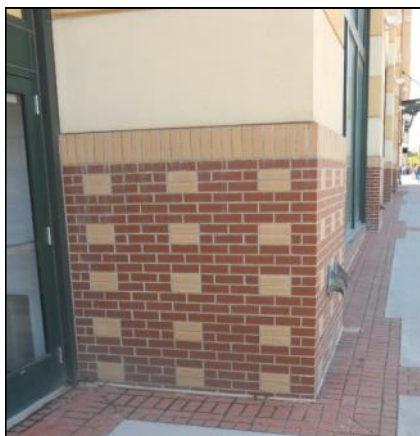
Brick, stone and other durable materials are required on the first floor of buildings.
