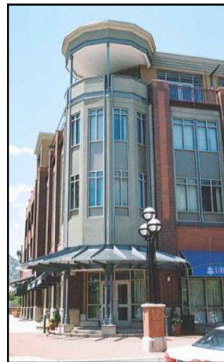
This building uses a rounded corner to address the intersection.
