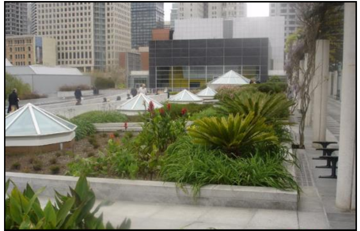
This rooftop garden helps reduce energy costs, reduces storm water runoff and provides places for people to gather.
