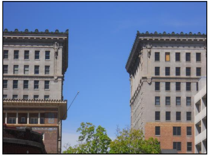
Prominent cornices, belt courses, and a rhythm of voids (windows) to solids (walls) are included on the sides of these buildings that are not adjacent to a street but are still visible from public spaces.
