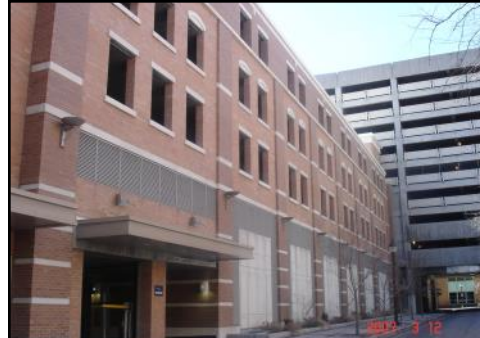
The parking structure in the foreground is designed with a rhythm of openings and building materials that complement the building. This parking structure is wrapped with office space adjacent to the street. The parking structure in the background does not reflect the desired design concepts.
