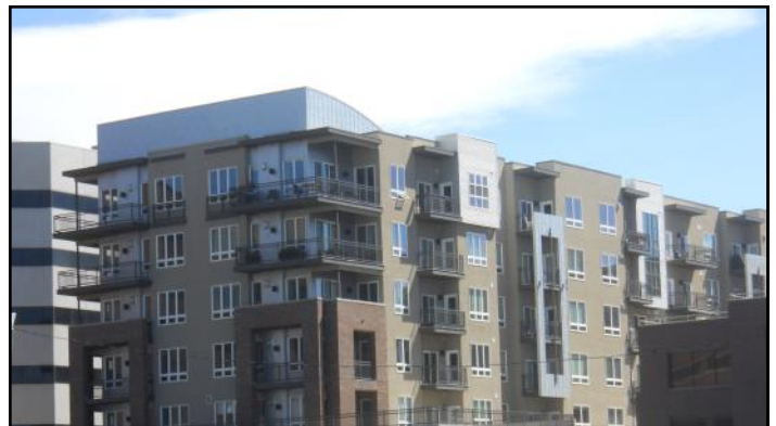
Breaks in wall planes, balconies, change in material, projections and bays add visual interest to the back and side of this building.
