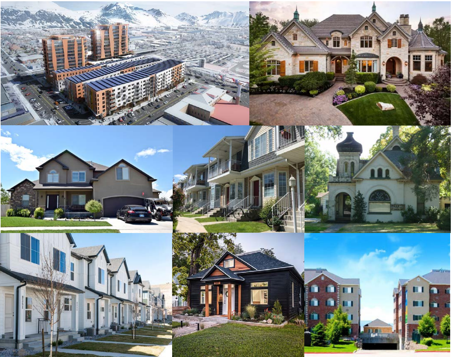
a variety of housing sizes, types, styles, and price points across Provo
