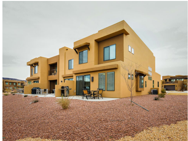
WCWCD is targeting a water allocation of 0.59 acre feet per year for new equivalent residential connections (ERUs).
