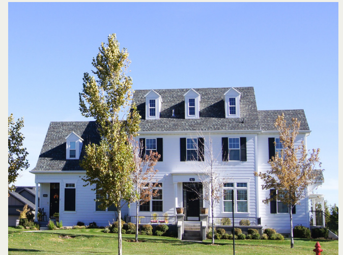
This home in South Jordan includes multiple units and is designed in a way that looks like a single-family home.
