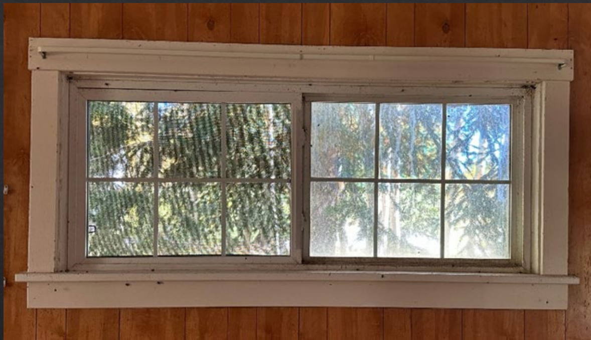
Measurements on existing vinyl windows.
