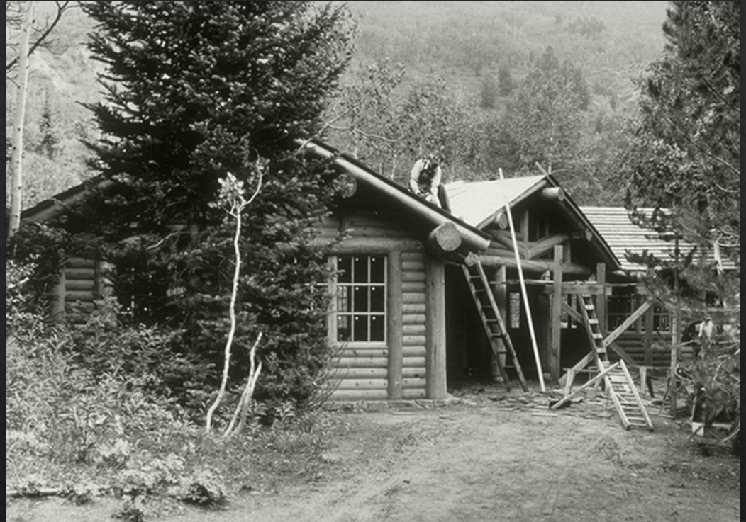
Spruces Pavillion being built in the 1930s
