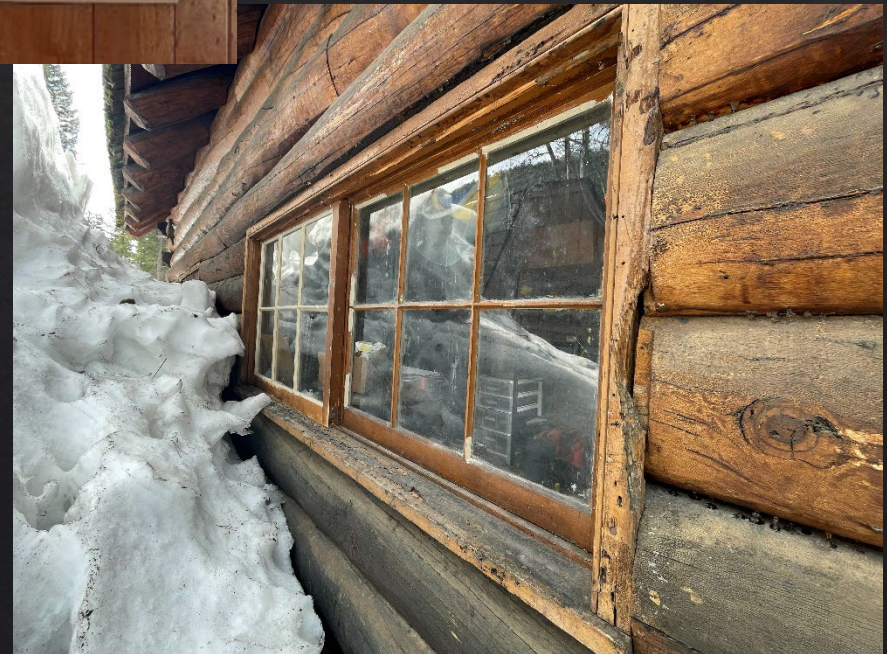
Example from another building with original windows.
