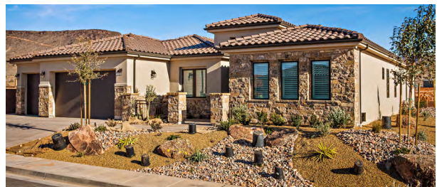
This 5,000 sq. ft lot in Southern Utah can still accommodate a single-family home and landscaping.
