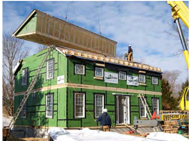
This modular home was created offsite and then assembled on the owner’s property. Image provided by New World Home.
