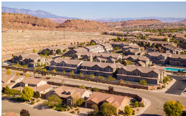
These townhomes in Southern Utah have a private alley that provides access to parking in back of the home.
