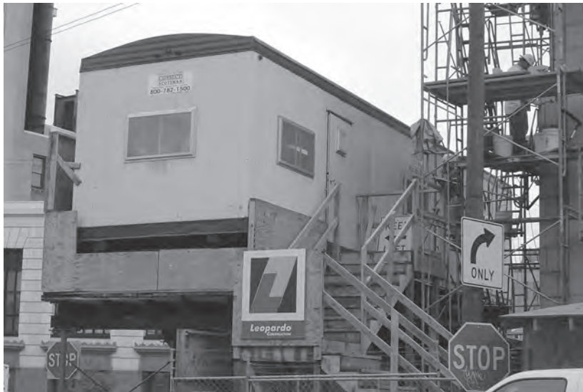
temporary construction field office
